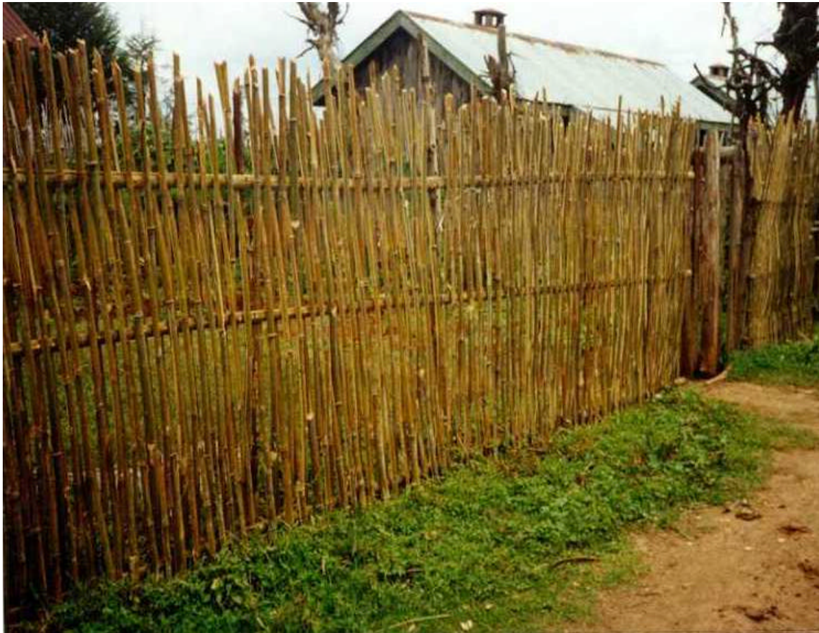
Plate 7: A newly constructed bamboo fence at Timboroa
